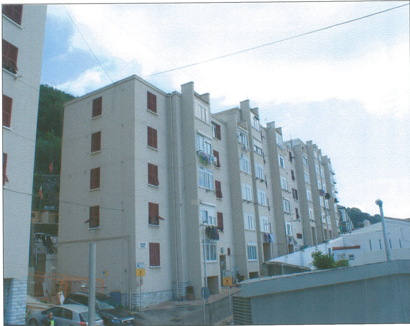
View as Existing
